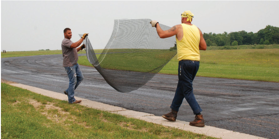
A GlasGrid mesh was also used over the cracks for additional reinforcement.
